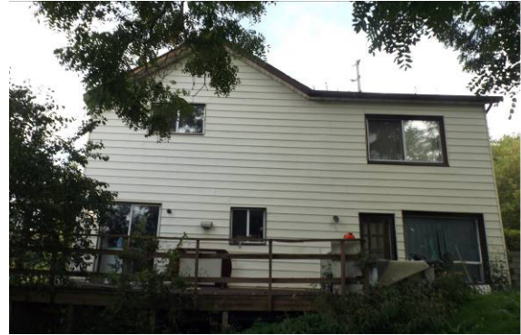
Figure 19. South side. Rear addition is not original. None of the openings are original.
