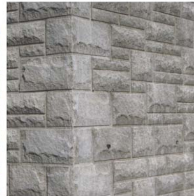
CONCRETE WALL TEXTURE ALONG NASHVILLE RD
