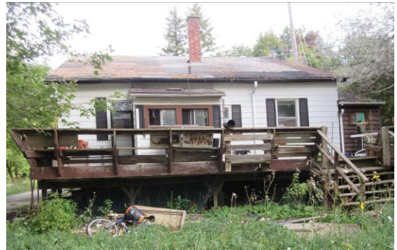
Figure 10. Rear (South) side. The deck and the shed additions at centre and right are not original.
