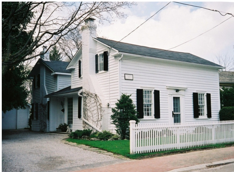
Figure 43. 30 Colbourne Street, Thornhill-Vaughan, showing rear addition from circa 1980. The addition is highly complementary to the original house..
