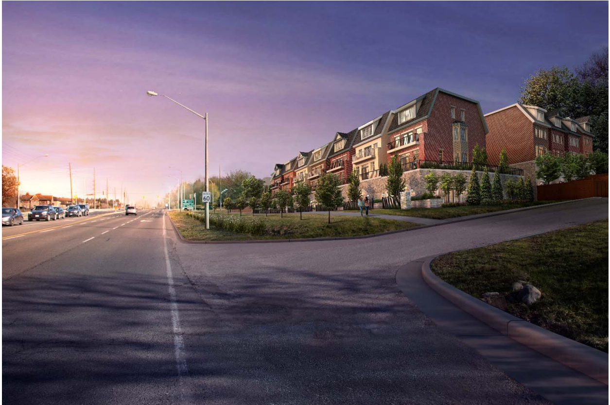
Image looking North from entrance to school property along Hwy 27
