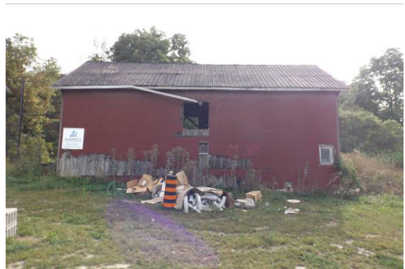
Figure 28. West side of the barn.
