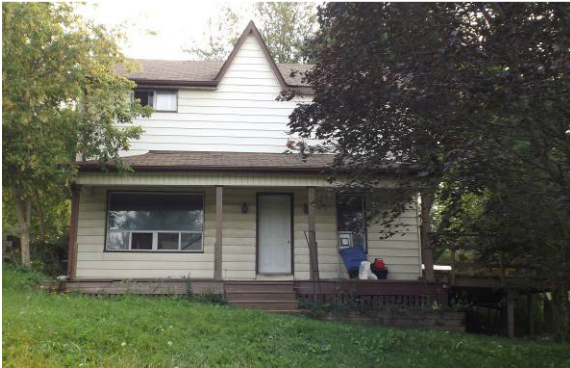
Figure 17. West (front) view of 99 Nashville Road. The house is set perpendicular to Nashville Road. None of the openings are original with the possible exception of the right-hand window on the ground floor.
