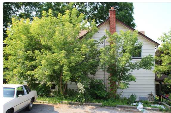
Figure 21. North side. None of the openings on this side are original.
