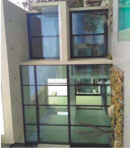
4 WINDOW WALL SYSTEM WINDOW WALL SYSTEM WITH CHARCOAL GREY MULLIONS AND CLEAR GLAZING
