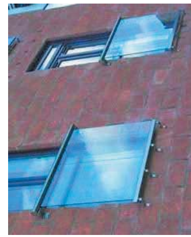
8 SANDBLASTED GLASS AND ALUMINUM RAILING GLASS AND ALUMINUM RAILING WITH SANDBLAST GLAZING
