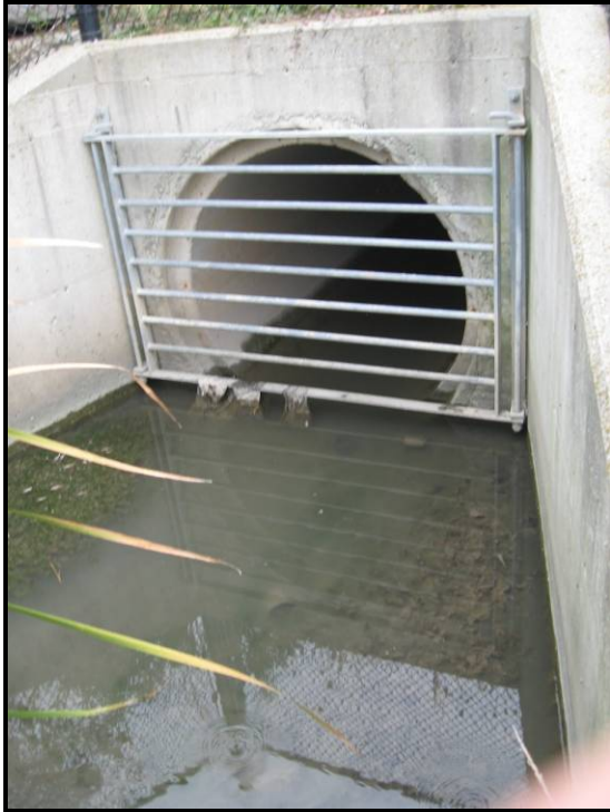
Photo 1. Outlet of SWM pond into Tributary B
