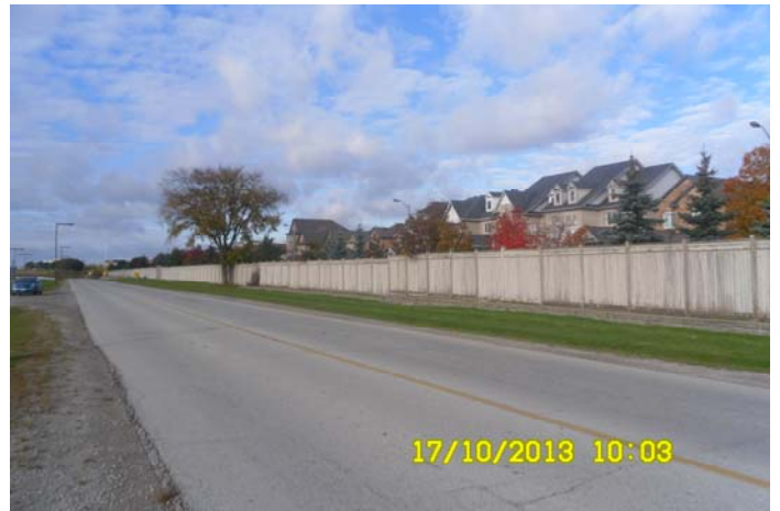
Photo 8: A view of northern portion of the Site looking west. Note the adjacent residential subdivision to the north.
