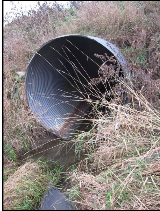
Photo 2. Culvert at Major Mackenzie Drive – Tributary A
