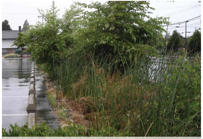
Figure 5.8: Bio-filtration with wet meadow type planting - Mt. Vernon WA, USA
