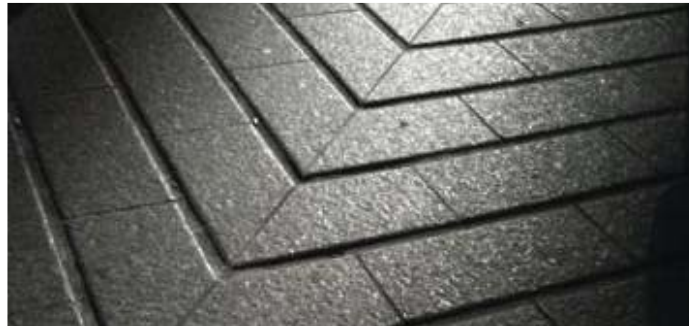
Figure 5.19: Tactile grooved pavers for use at pedestrian ramps
