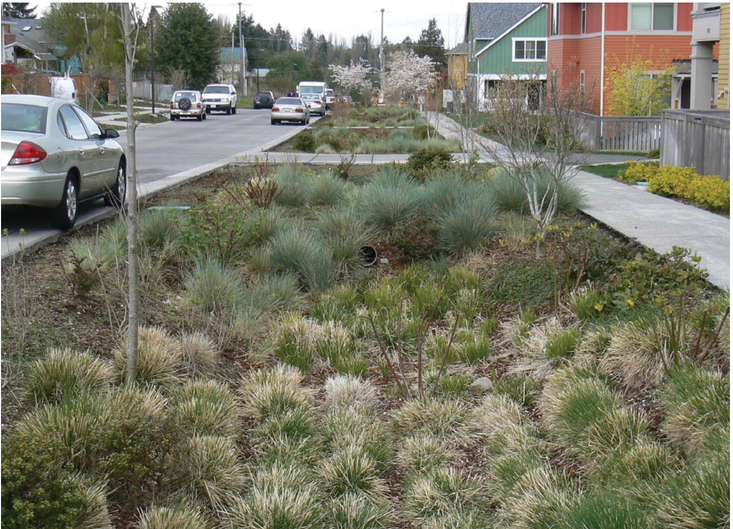
Figure 5.9: Bio-filtration swale - High Point, Seattle WA, USA
