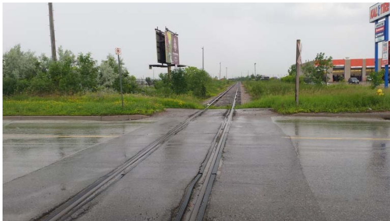
Photo 8 – The rail spur located immediately adjacent to the north of the eastern end of Part B of the Site, looking east.
