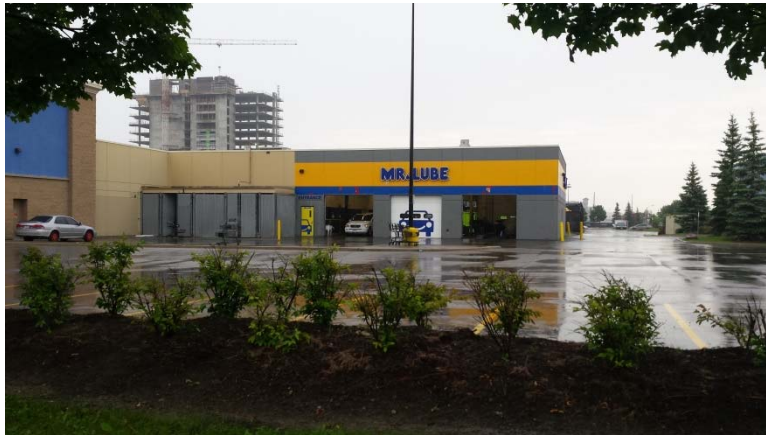
Photo 3 – View of the off-Site Mr. Lube, located at 100 Edgeley Boulevard, looking south from the Site.
