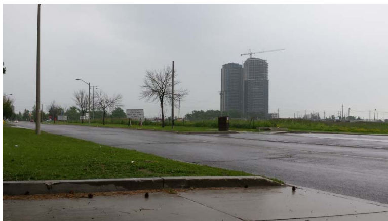
Photo 4 – View of the eastern end of Part A, looking southeast from the northern side of Portage Parkway.
