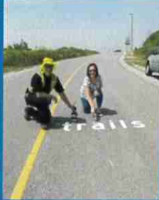
NMRP Road Paving
