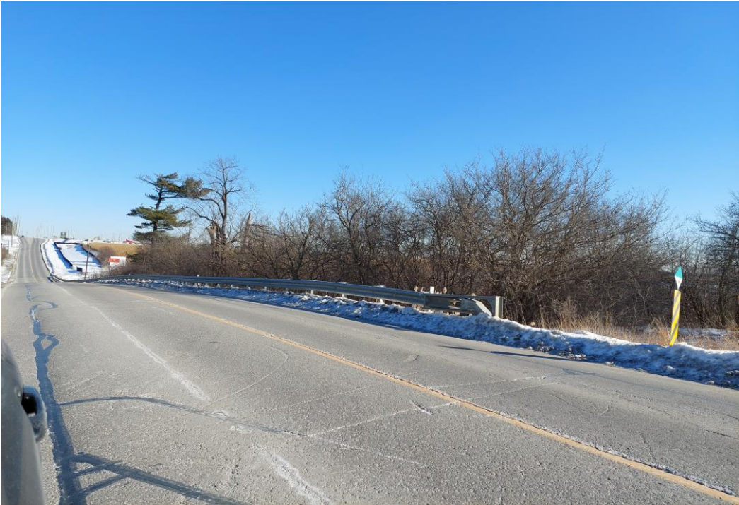
Photo 5: Teston Road at Sta. 2+600, Looking East
