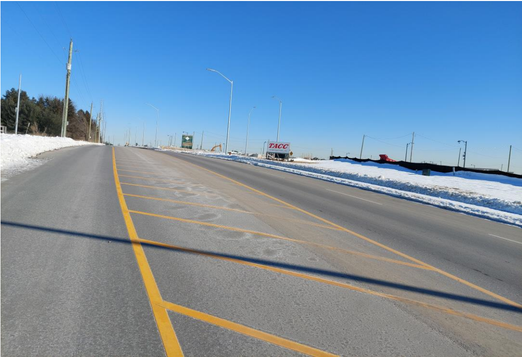
Photo 7: Teston Road at Sta. 2+950, Looking East
