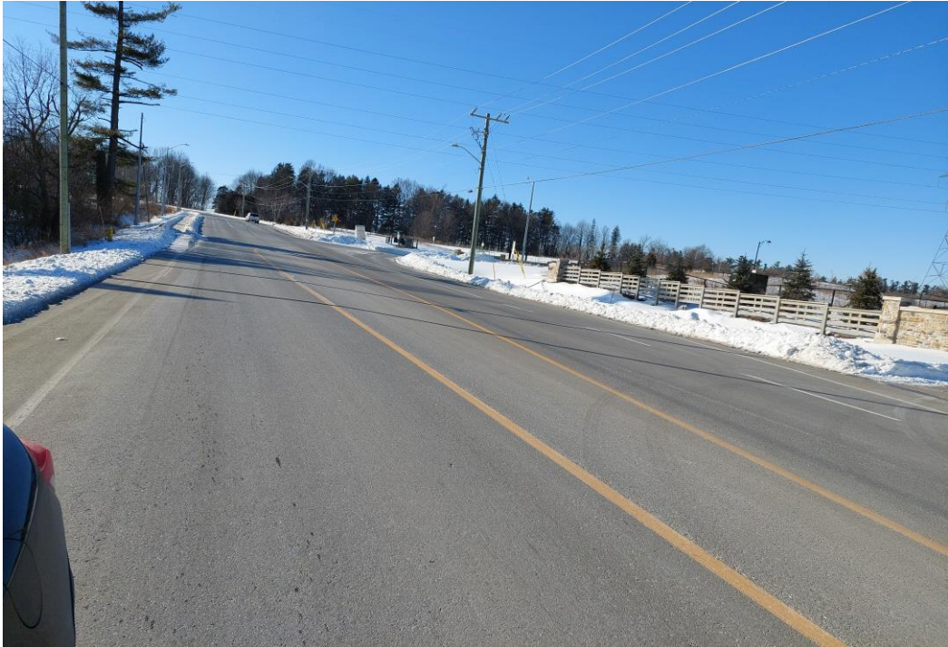
Photo 2: Teston Road at Sta. 1+120, Looking West
