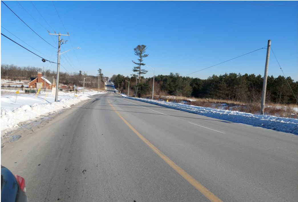
Photo 1: Teston Road at Sta. 1+000, Looking East
