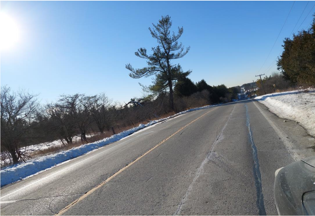
Photo 6: Teston Road at Sta. 2+600, Looking West
