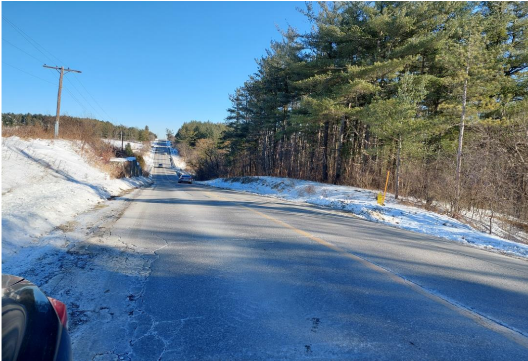
Photo 4: Teston Road at Sta. 2+050, Looking East
