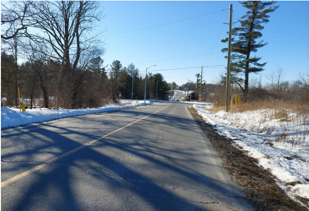
Photo 3: Teston Road at Sta. 1+450, Looking West
