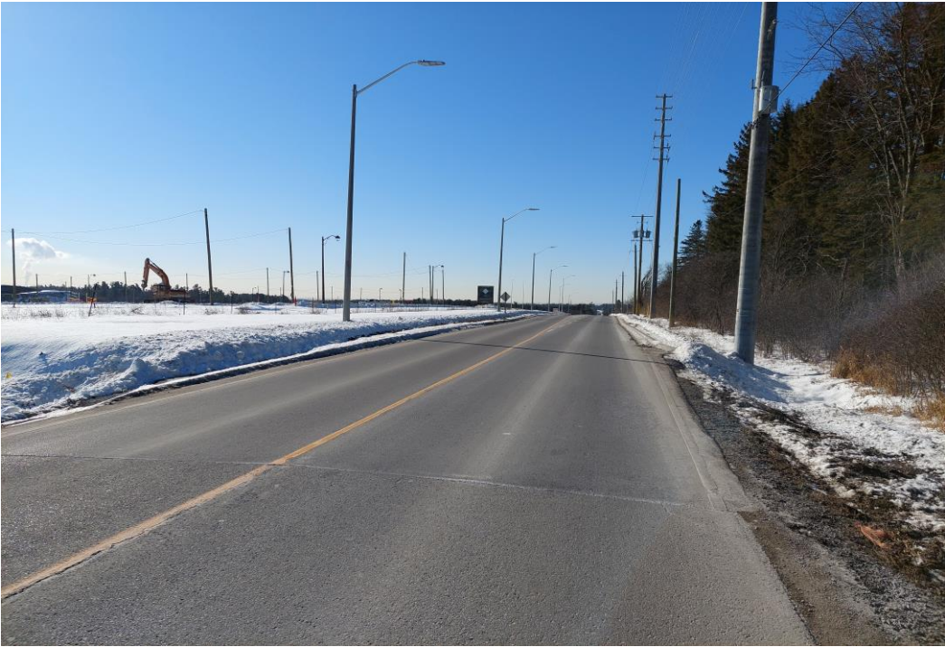
Photo 8: Teston Road at Sta. 3+175, Looking West
