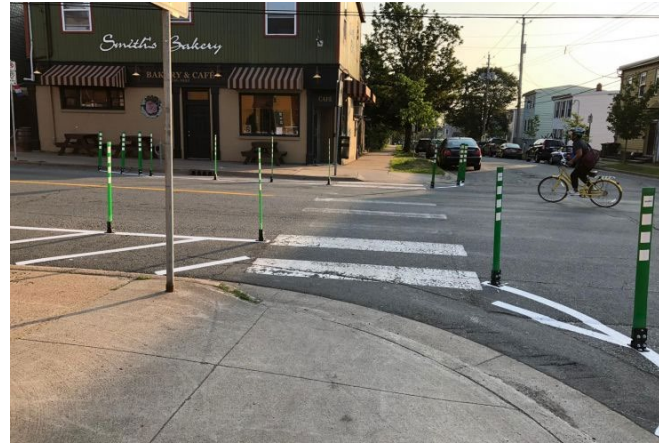
Temporary Curb Extensions
