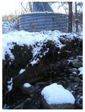
Photo 10. Erosion along northern bank of Black Creek near Hydro One tower foundation (ES10)
