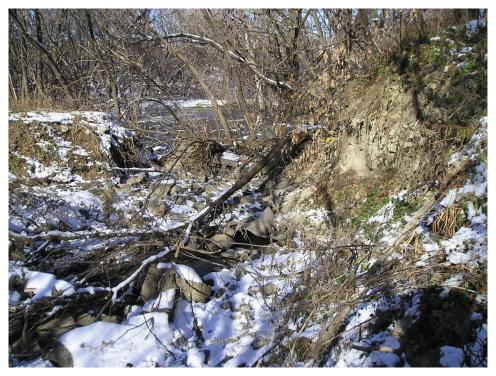
Photo 18. Breached access road berm, destroyed culverts and eroded valleyside (ES18)
