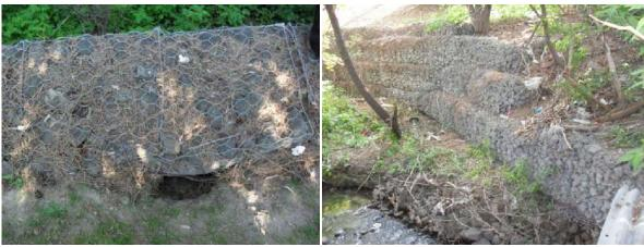
Figure 3 🛧 Void behind the wall
