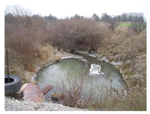
Photo 6. Scour pool below perched culvert and eroding road embankment (ES6)
