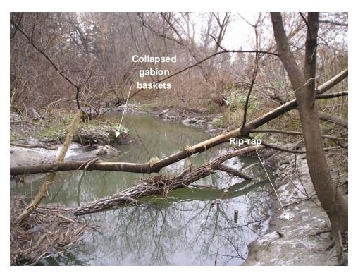
Photo 3. Collapsed gabion baskets and rip-rap (ES3)
