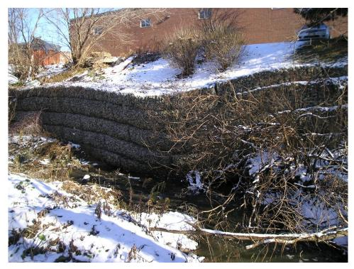
Photo 17. Undermined gabion retaining wall collapsing into channel (ES17)
