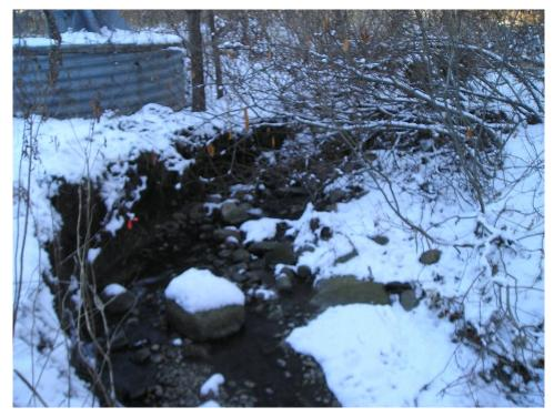
Photo 12. Degradation and bank erosion at footing of hydroelectric tower (ES12)
