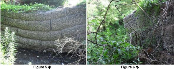
Figure 5 🛧 Deformed area of the wall
