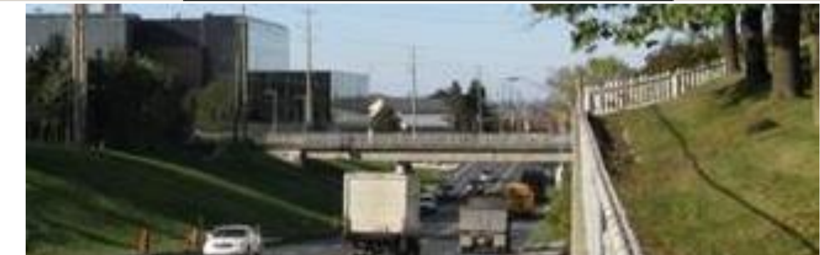
Underpass example on Major Mackenzie Drive east of Keele Street
