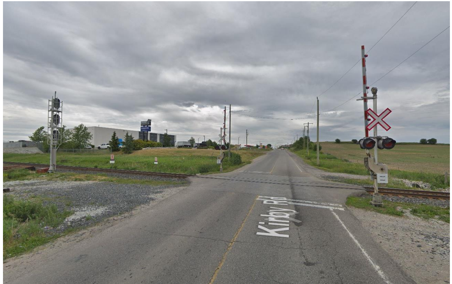
Looking east at Barrie GO Rail Corridor At-Grade Crossing
